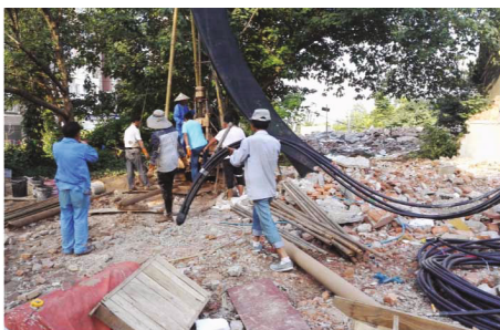
FIGURE 5: Installation of vertical heat exchanger.
