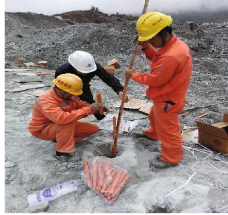
FIGURE 4: Air interval charging.
