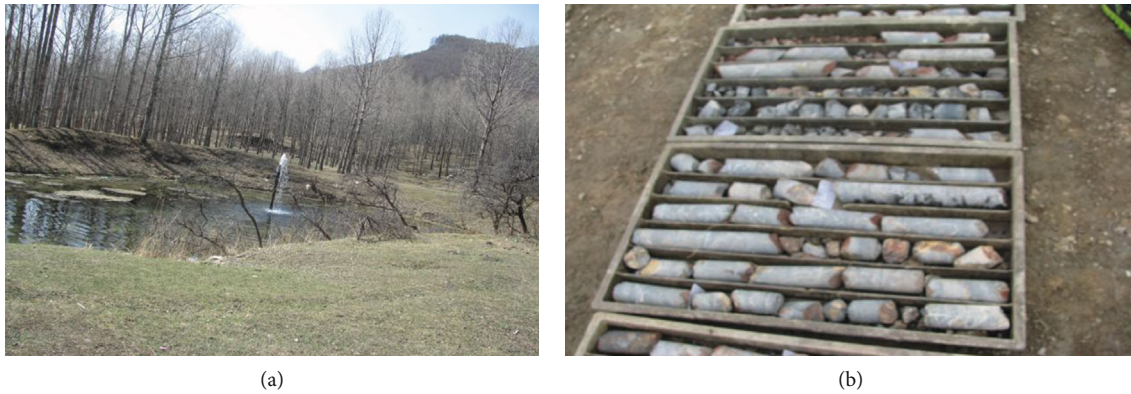
FIGURE 16: Photo of the groundwater flowing borehole behind the dam (a) and core drilled on site (b).
