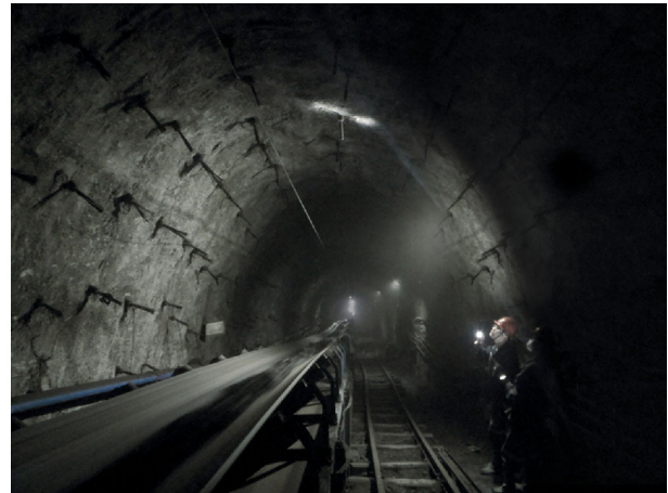
FIGURE 12: Image of the ACC support scheme eight months after tunnel construction.
