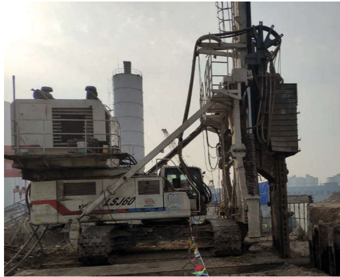
FIGURE 2: TRD machine in working.
