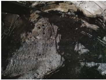
FIGURE 11: Probe hole after grouting.
