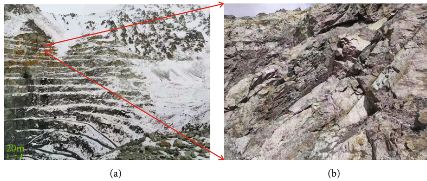
FIGURE 1: Description of the rock mass structural characteristics in the eastern open pit slope of Beizhan iron mine. An obvious rock bridge structure can be observed from the outcrop.
