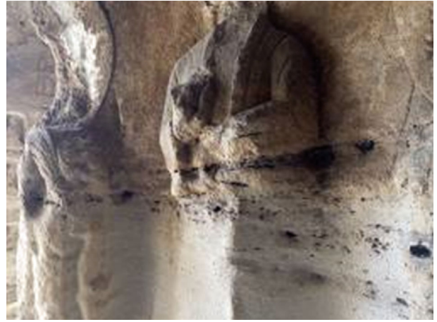
FIGURE 1: Local hole-like weathering in sculpture layer in Yungang Grottoes.
