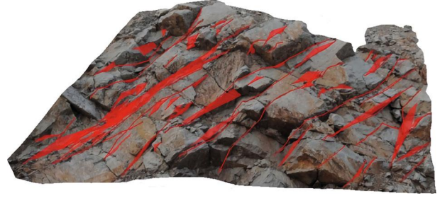
FIGURE 1: Natural cracks on the tunnel face onsite.
