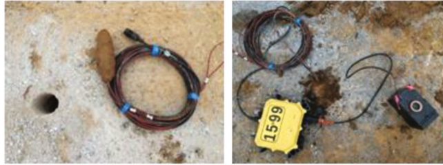
FIGURE 3: Equipment installation at site monitoring points.
