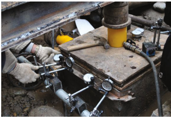
FIGURE 3: Field shear test.
