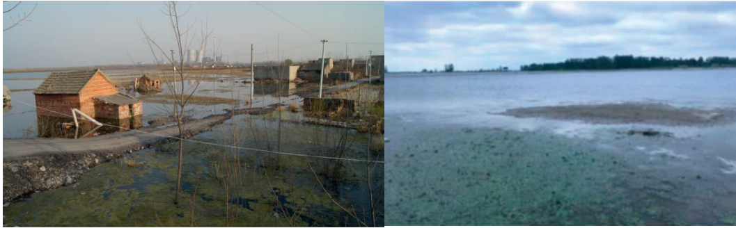
FIGURE 1: High-water-level coal mining subsidence area.
