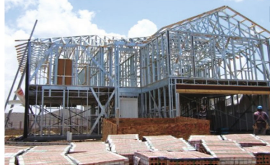
FIGURE 1: Light steel-wood-plastic structure building.
