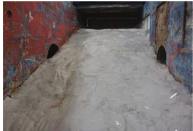
FIGURE 9: The paving of sliding belt materials.
