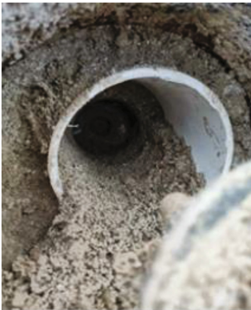
(c) Third excavation
