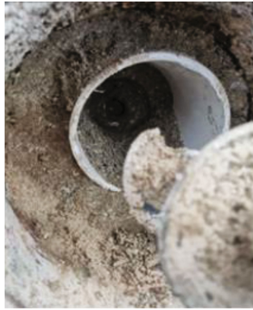
(b) Second excavation
