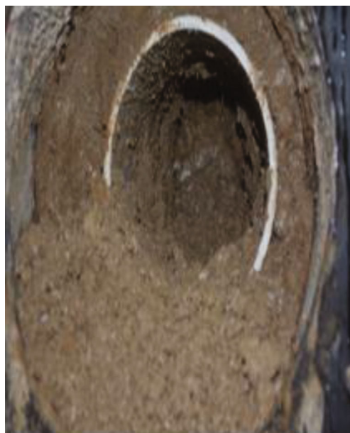
(h) Eighth excavation
