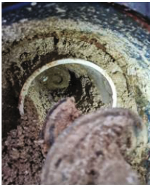
(e) Fifth excavation
