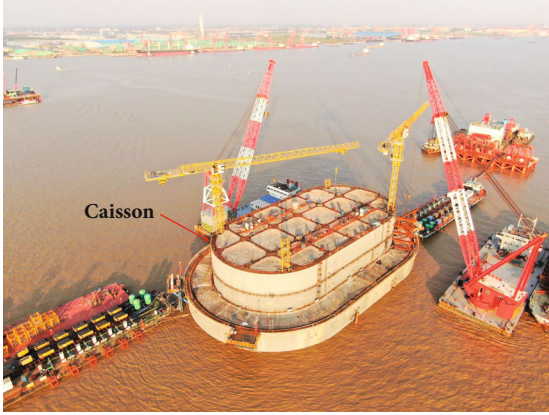
FIGURE 2: Caisson under construction.
