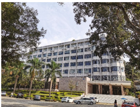
FIGURE 3: The seven-story classroom building under investigation.
