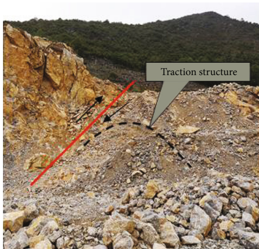
FIGURE 3: F1 fault crossing the slope.
