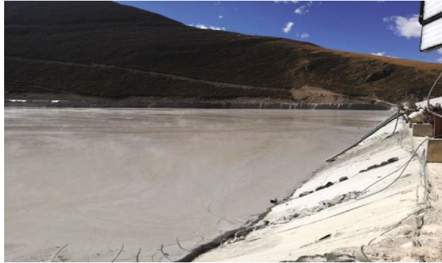
FIGURE 1: Tailing beach surface in the initial dam.
