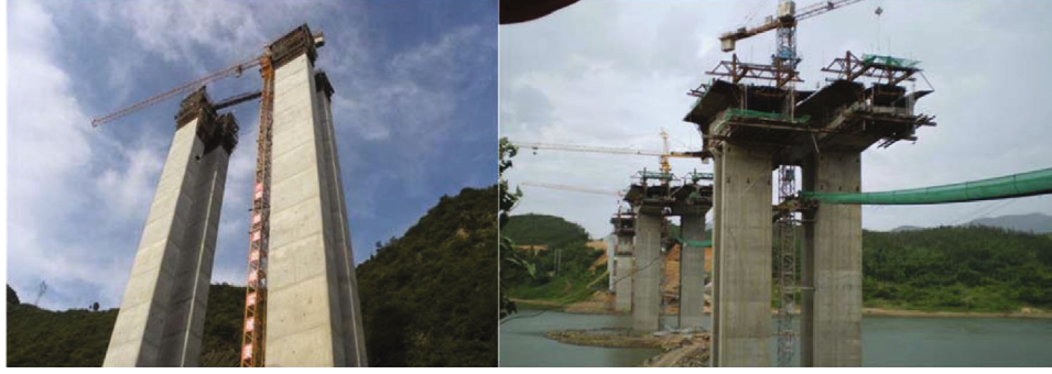
FIGURE 3: Double-limb thin-walled pier under construction in the river-crossing project.
