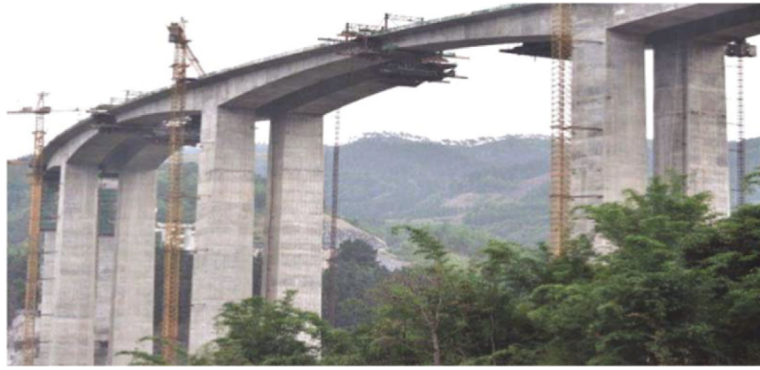
FIGURE 2: Single-limb thin-walled pier under construction.
