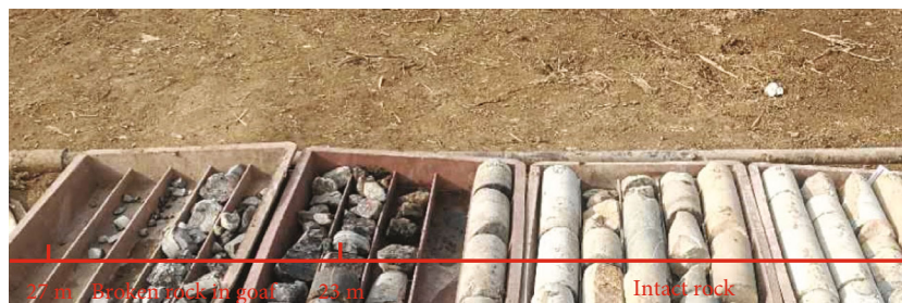
FIGURE 13: H-3 core before grouting treatment.
