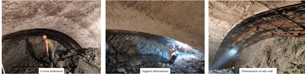
FIGURE 3: Tunnel deformation.
