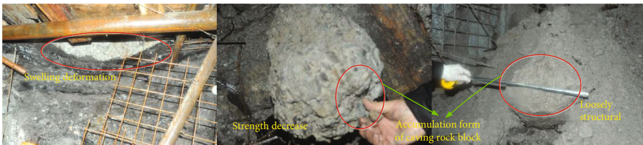
FIGURE 2: The morphological characteristics of falling rocks.
