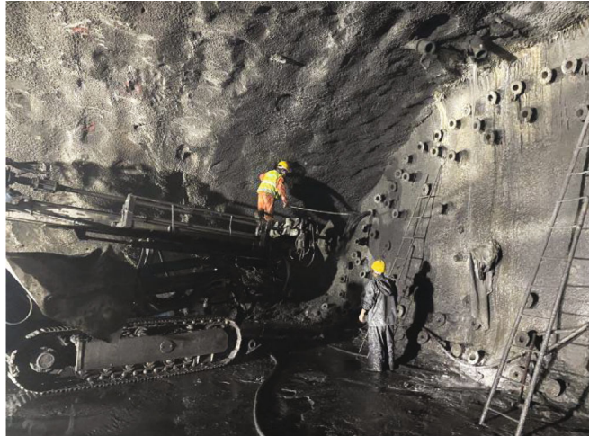
FIGURE 13: Use sulfoaluminate cement for grouting hole B28.
