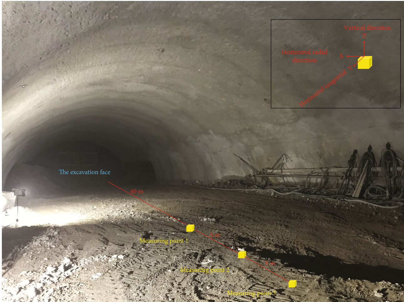
FIGURE 2: Layout of bottom plate measuring points.
