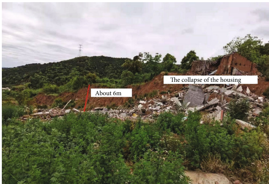
FIGURE 8: Fault zone at the back edge of the landslide. The trailing edge of the collapse zone extends from north to southwest, with a maximum depth of 6 m and a total length of approximately 210 m.
