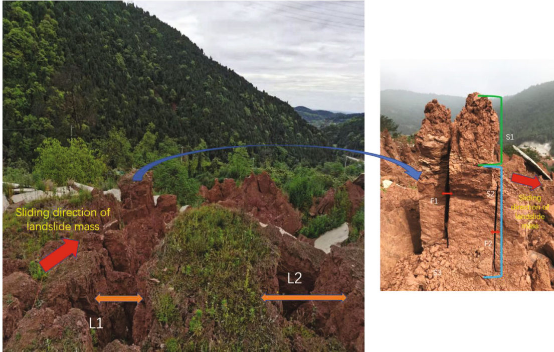
FIGURE 2: Landslide area surface photographed in different seasons. The picture on the left was taken on September 1, 2020. The picture on the right was taken on March 2, 2021. L represents the almost north–south fracture, F represents the almost east–west fracture, and S represents weathered red-bed soft rock.
