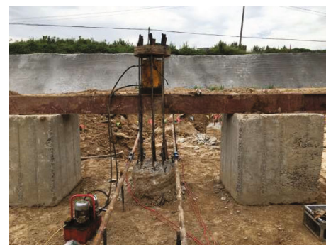
FIGURE 6: Field vertical pulling test.
