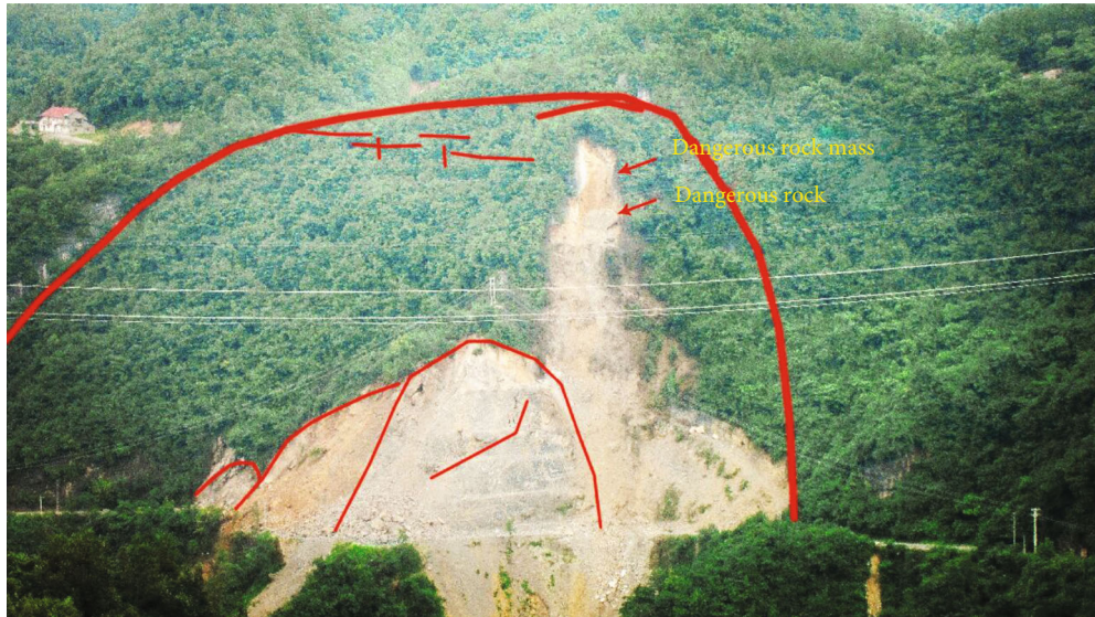
FIGURE 3: Overall view of Tanziyan landslide.
