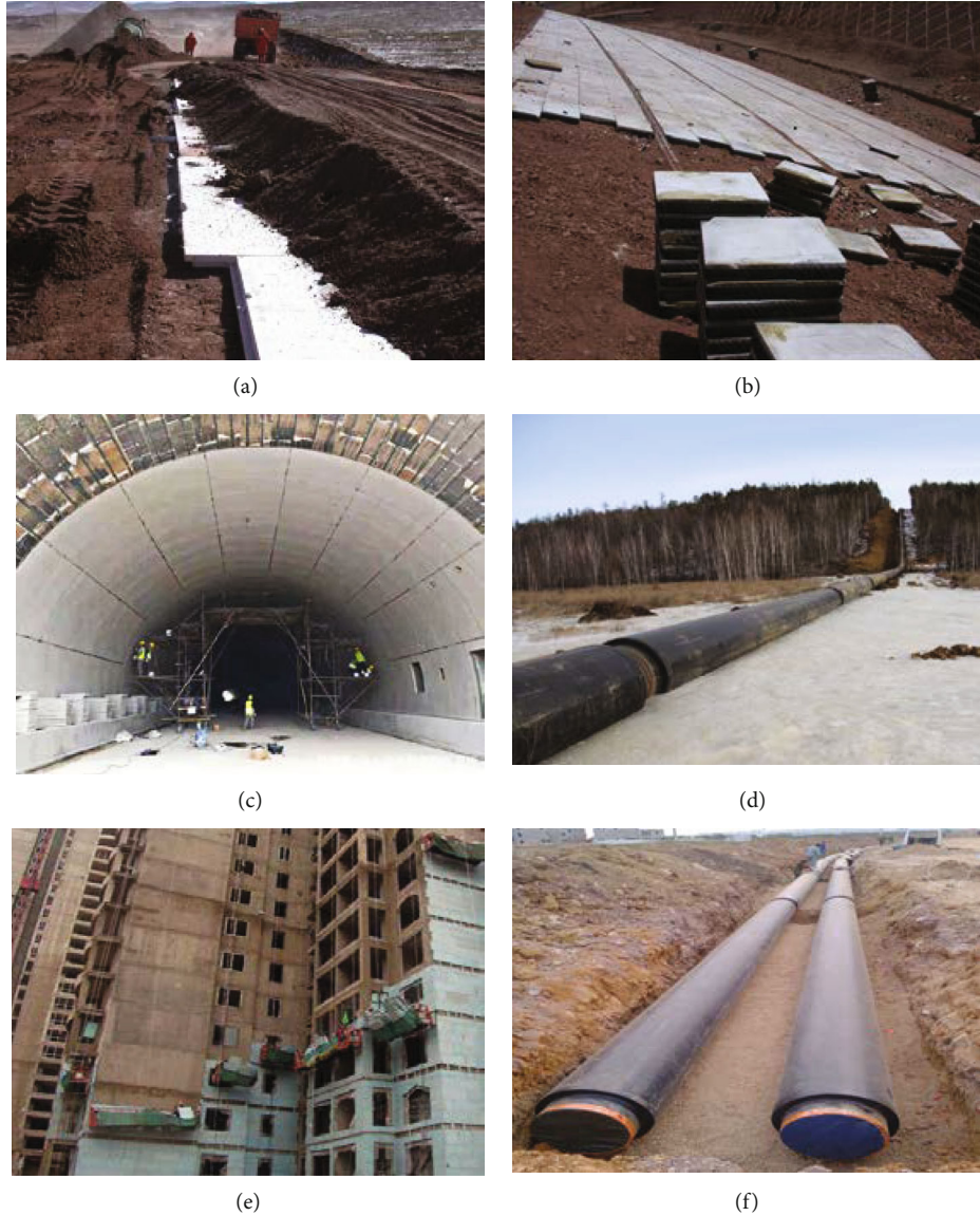
FIGURE 1: TIMs used in (a) roadway embankment, (b) cutting slopes, (c) tunnels, (d) oil pipelines, (e) buildings, and (f) municipal pipelines in cold regions.
