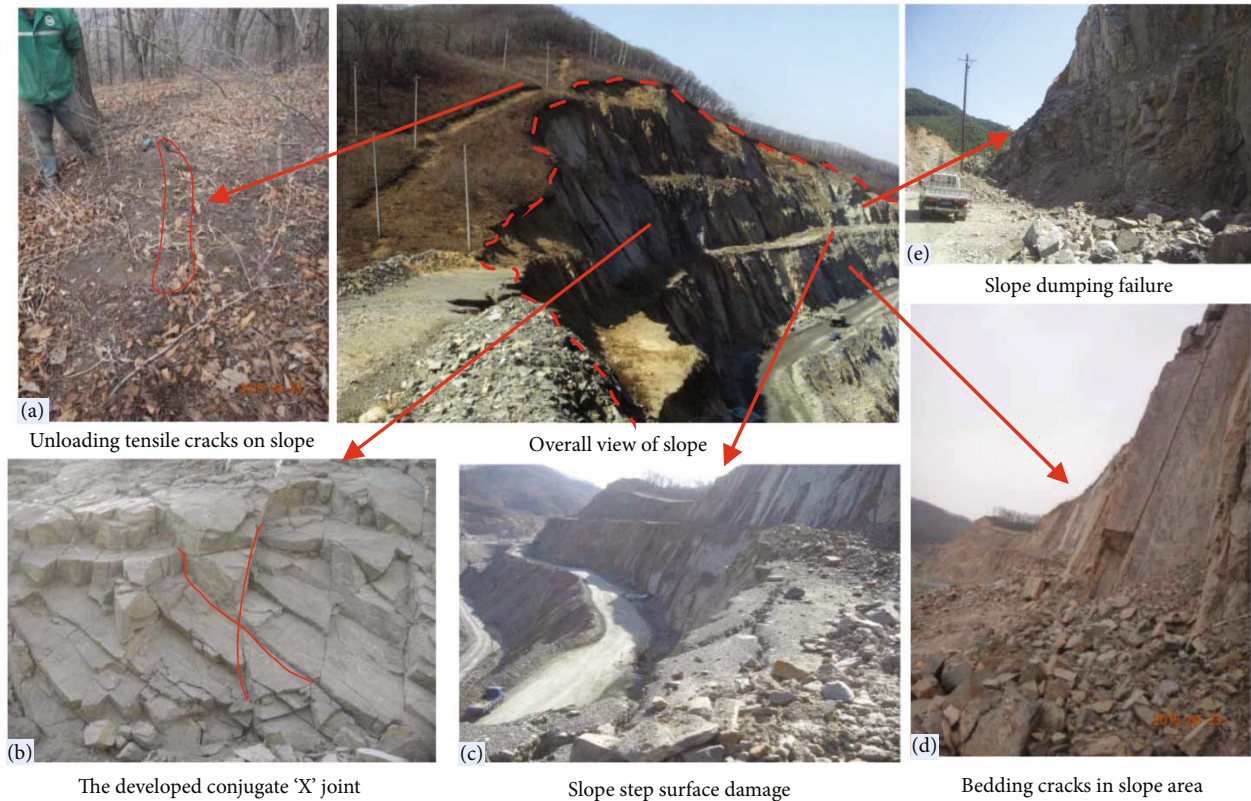
FIGURE 6: Deformation and failure diagram of the slope.
