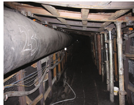
FIGURE 12: The stable reused roadway surrounding rock after roof presplitting.
