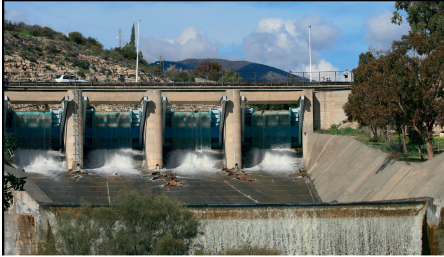
FIGURE 1: Panoramic view of ladder-shaped spillway.
