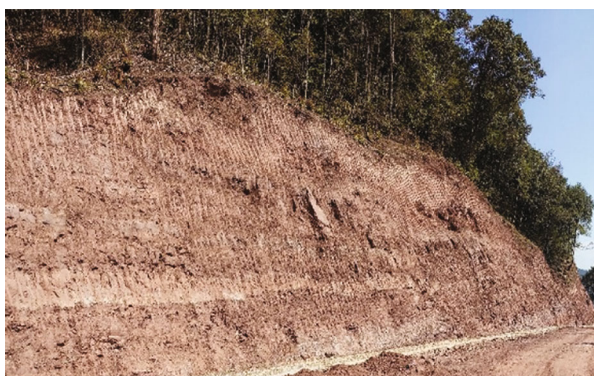
(a) Field rock survey
