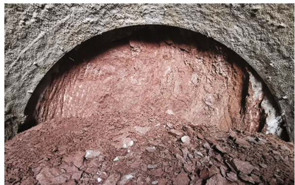
(b) In-tunnel survey
