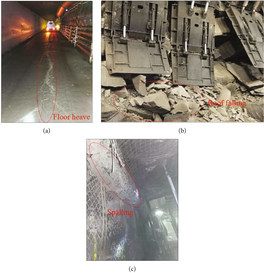
FIGURE 2: Roadway deformation and failure diagram.
