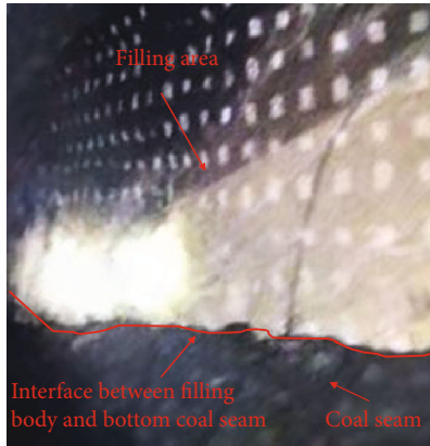
FIGURE 13: Filling and excavation effect of the project site.
