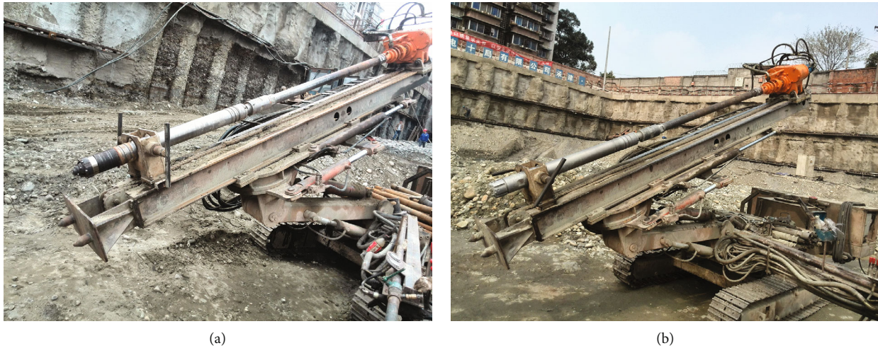
FIGURE 16: Drilling experiment field: (a) percussion compact bit drilling experiment; (b) reverse circulation bit drilling experiment.
