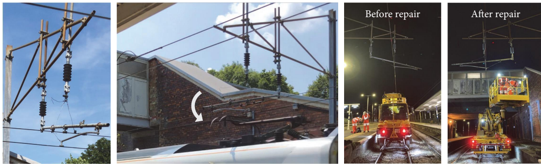
FIGURE 34: Detached nose dropper leads to registration tube falling at far end.
