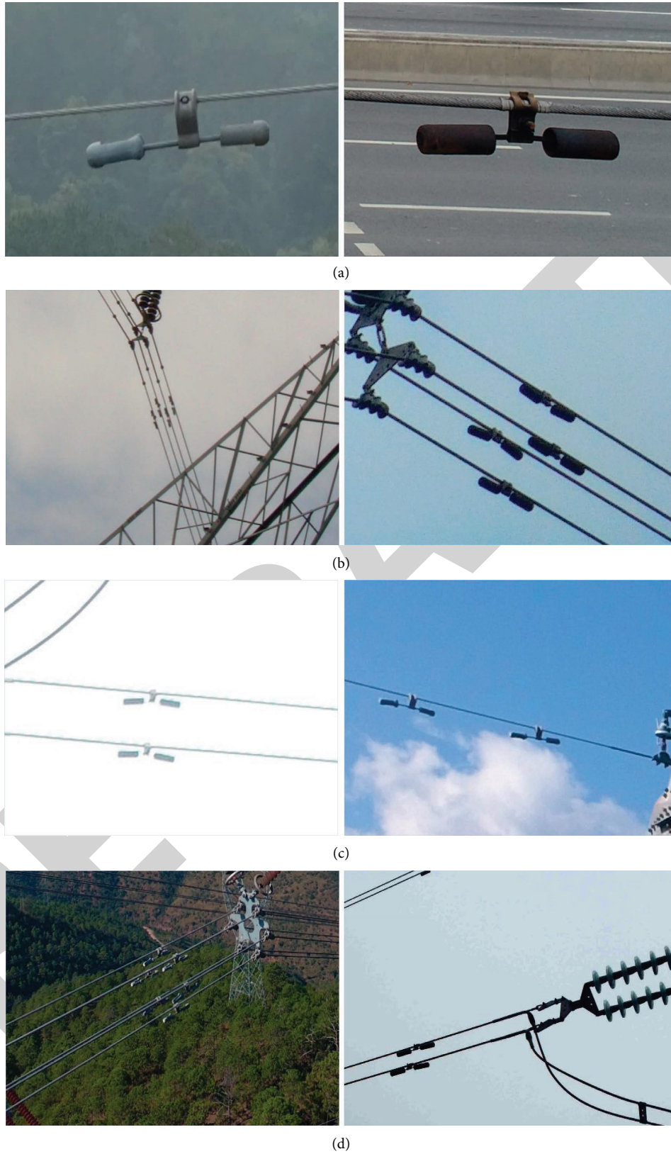
FIGURE 9: Typical images of antivibration hammers divided into four common conditions: (a) two common types of antivibration hammers, (b) two different sizes of antivibration hammers, (c) two different lighting conditions of antivibration hammers, and (d) two different backgrounds of antivibration hammers.
