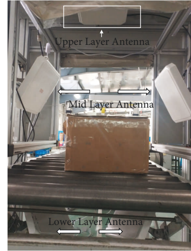
FIGURE 5: RFID reader actual antenna deployment.
