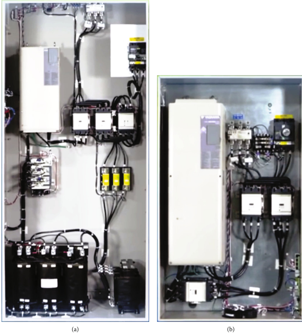
FIGURE 12: (a) DC link-based drive. (b) Matrix converter-based drive (courtesy: Yaskawa Inc.).
