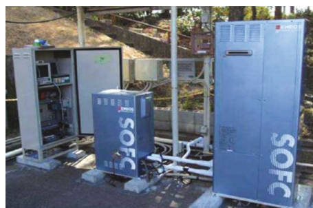
FIGURE 14: Residential CHP system based on SOFCs, which was developed by Tokyo Gas, Osaka Gas, and Eneos in Japan [21].
