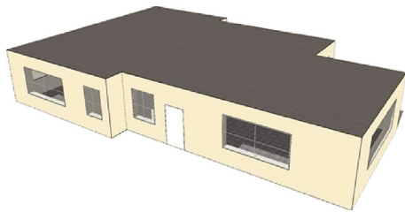
FIGURE 3: General view of the building.
