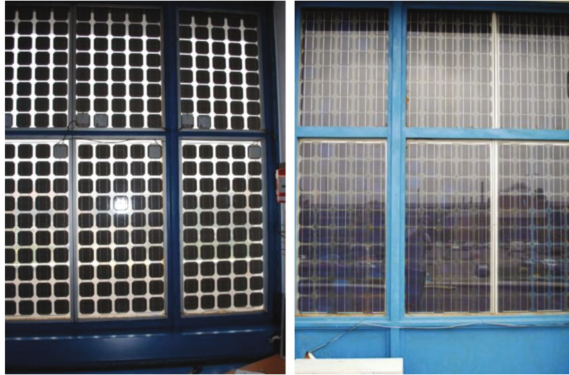
FIGURE 3: BIPV system developed within the laboratory of nanostructures, solar cells, and PV systems from the Department of Physics, Faculty of Applied Sciences, Polytechnic University of Bucharest (inside/outside view).
