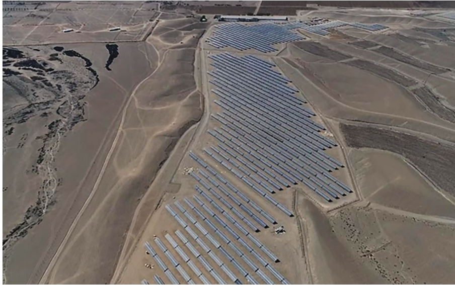
FIGURE 1: Valle Solar Oeste photovoltaic plant.
