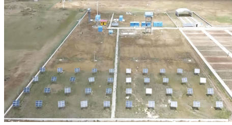
FIGURE 8: Photovoltaic panel site array view.
