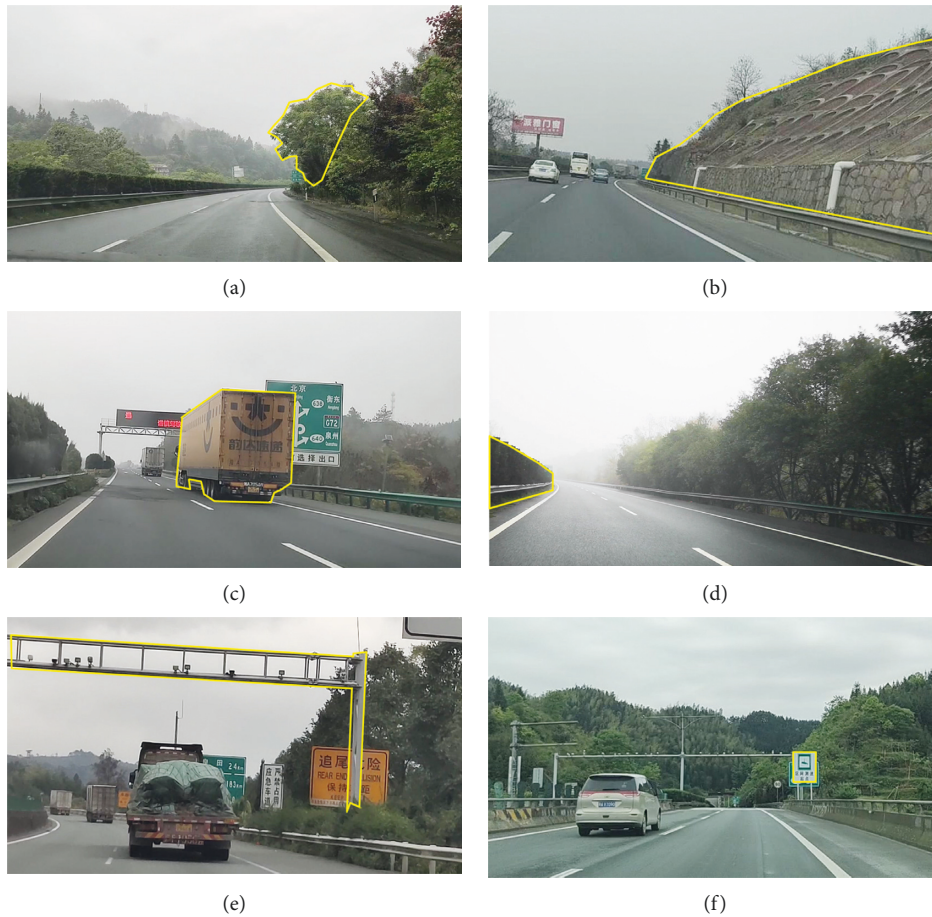
FIGURE 3: Illustration of occlusion factors (for details, refer to the text). (a) Plant occlusion. (b) Slope occlusion wall. (c) Dynamic occlusion of codirectional vehicles. (d) Occlusion from central divider. (e) Occlusion of monitoring facilities. (f) Occlusion of traffic signs.
