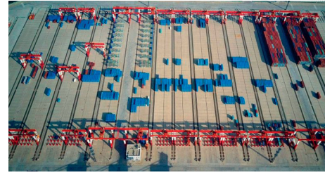
FIGURE 1: Twin ASC stacking blocks at Yangshan automated container terminal.
