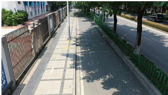
(5) Actual survey view of CuiZhu Road
