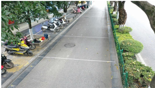
(3) Actual survey view of Jiefang East Road Section C
