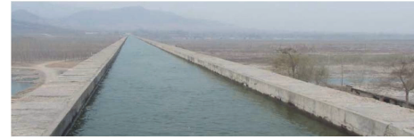
FIGURE 4: A single-pool canal in Yehe irrigation area.
