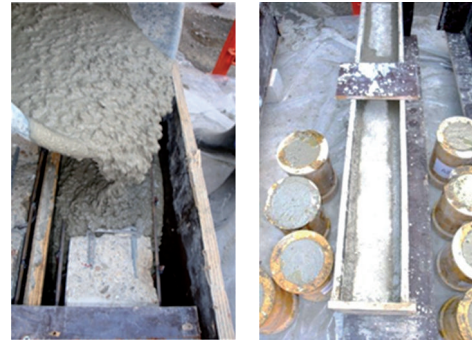
FIGURE 4: Formwork of the jacket and SCC pouring.
