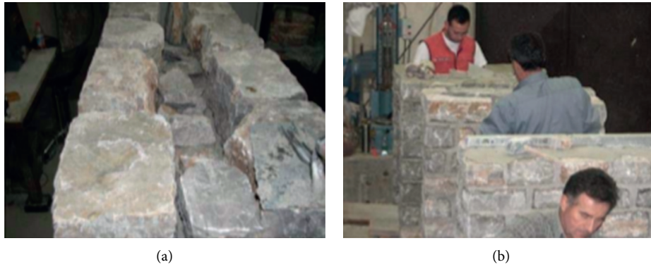
FIGURE 2: Construction of wall with no connecting stones [18].
